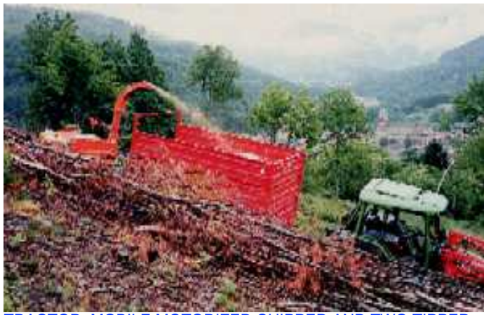
TRACTOR, MOBILE MOTORIZED CHIPPER AND TWO TIPPER-TRAILERS
