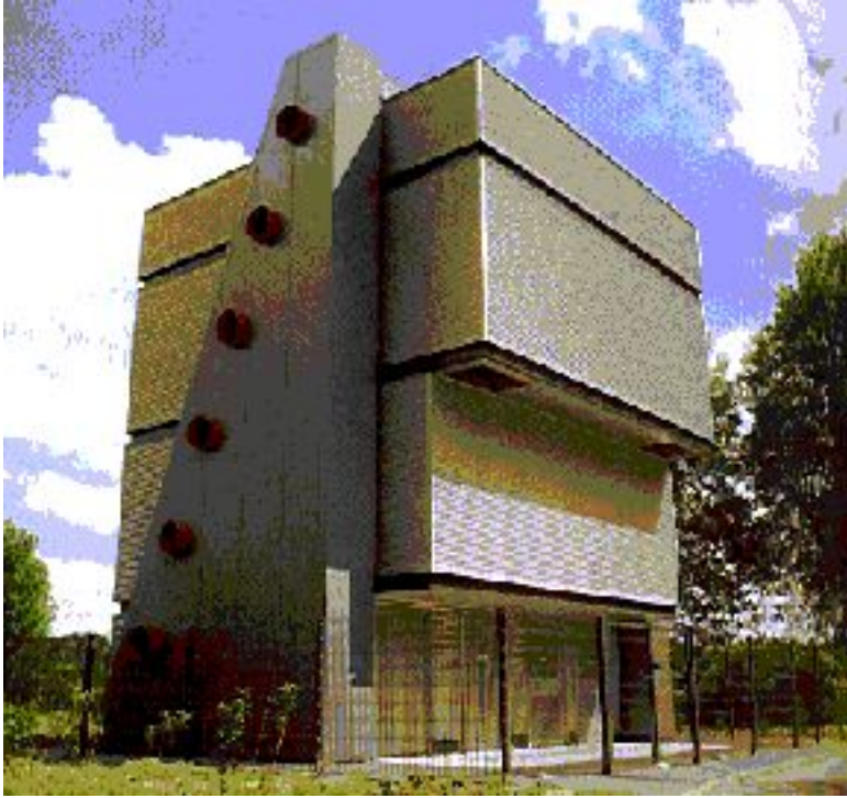
ARNHEM COGENERATION PLANT
